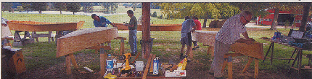
Students worked on building their wooden boats at the Tennessee Boat School in Big Sandy, Tenn. Major parts of the boats are pre-cut from plywood and oak.
